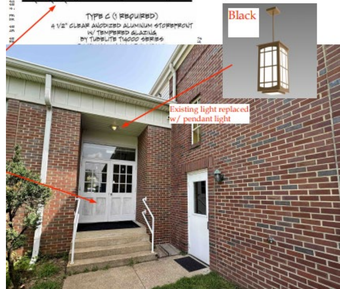
Figure 2 Secondary Elevation, northwest
