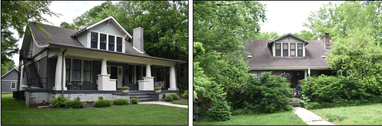
Figure 6-09. Left photo of Field No. BC-6 at 806 Barrow Court; view to the northwest. Right photo of the Field No. BC-11 at 814 Barrow Court; view to the west.
