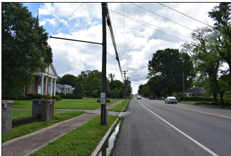
Figure 3-21. Streetscape photo showing west of Terrace Drive showing the north and south sides of W. 7 th Street; view to the east.
