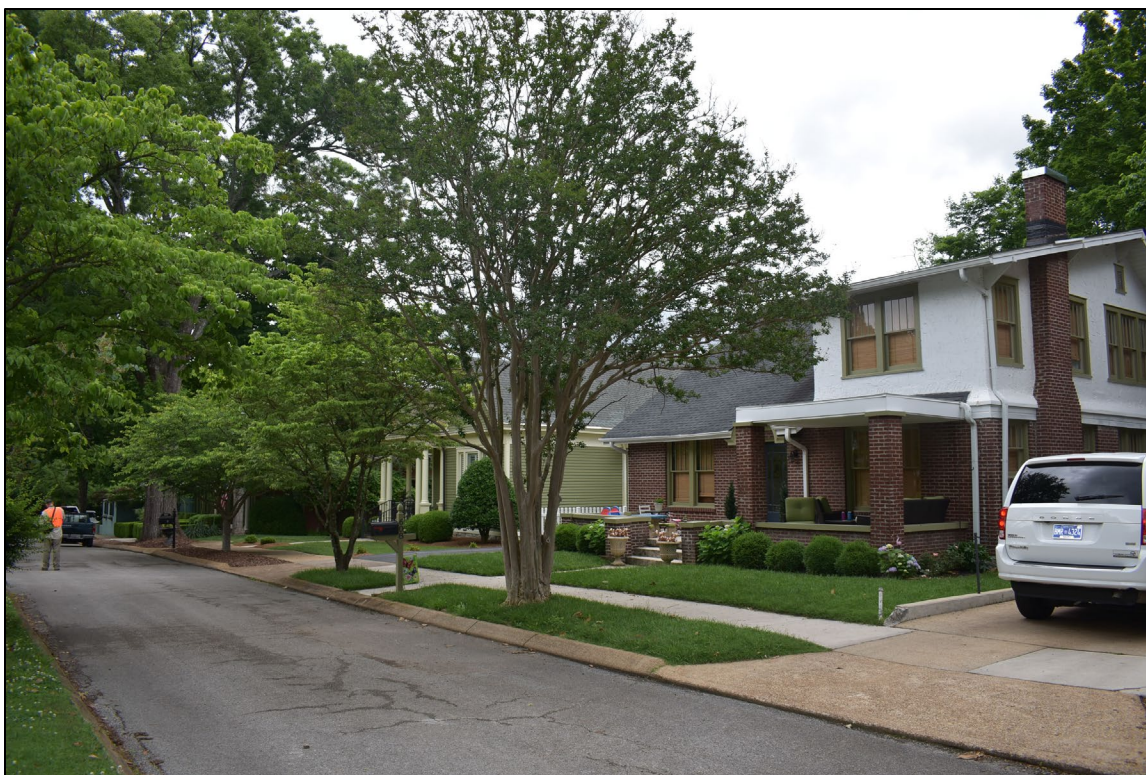
Figure 4-09. Streetscape of the east side of Mayes Place showing Field Nos. HS-52, HS-54, and HS-56 (left to right); view to the northeast.
