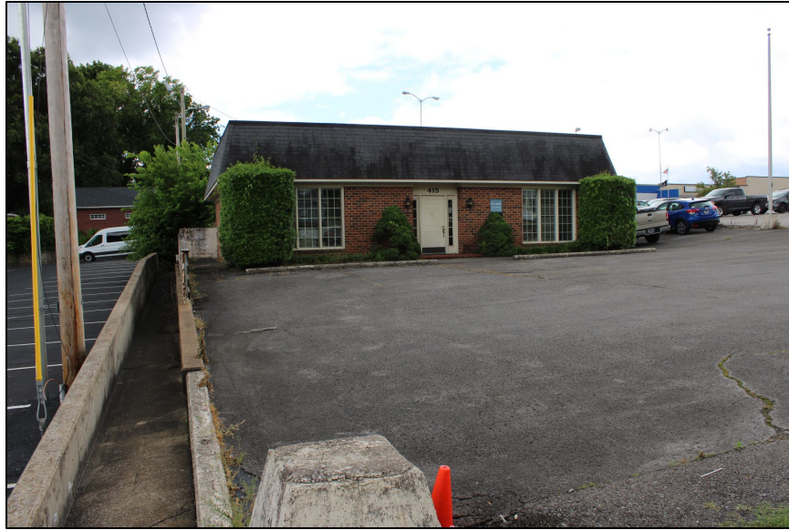
Figure 3-28. Photo of c. 1961 office building at 415 W. 7 th Street (Field No. HS-132); view south.
