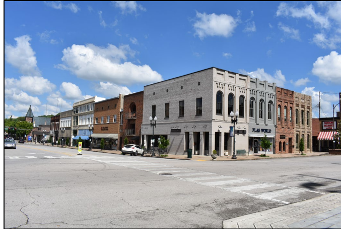
Figure 5-29. Streetscape photo with the right side showing 29-33 Public Square (Field Nos. HS-286, HS-287, and HS-288; left to right) in the northwest corner of the square and the left side showing 100-120 W. 7 th Street (Field Nos. HS-357, HS-258, HS-360, HS-363, HS-364, HS-365, and HS-368; left to right); view to the northwest.
