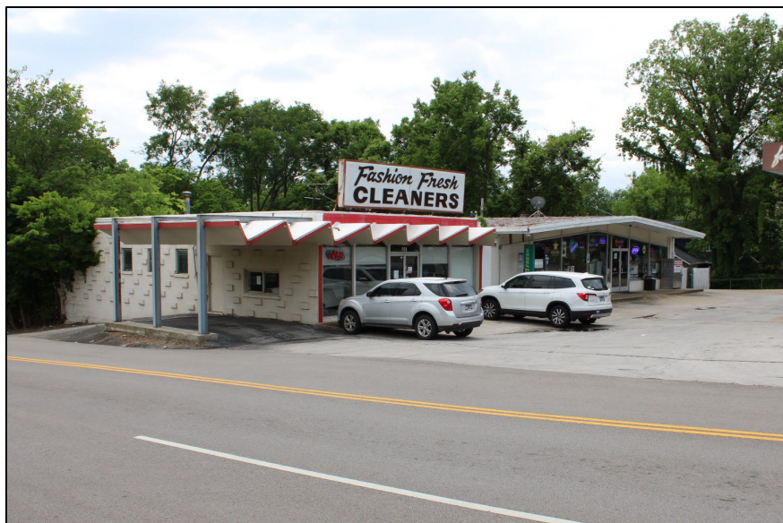
Figure 6-15. Photo shows 703 Trotwood Avenue (Field No. BC-4; left) and 701 Trotwood Avenue (Field No. BC-3; left); view to the southwest.
