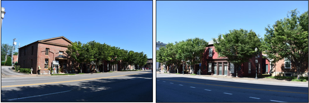
Figure 5-32. Streetscape photos of the west side of S. Garden in the NRHP boundary. Left Photo shows Field Nos. HS-302, HS-300, and HS-297 (left to right); view to the northwest. Right photo shows Field No. HS-297 with HS-298 in the right background; view to the southwest.
