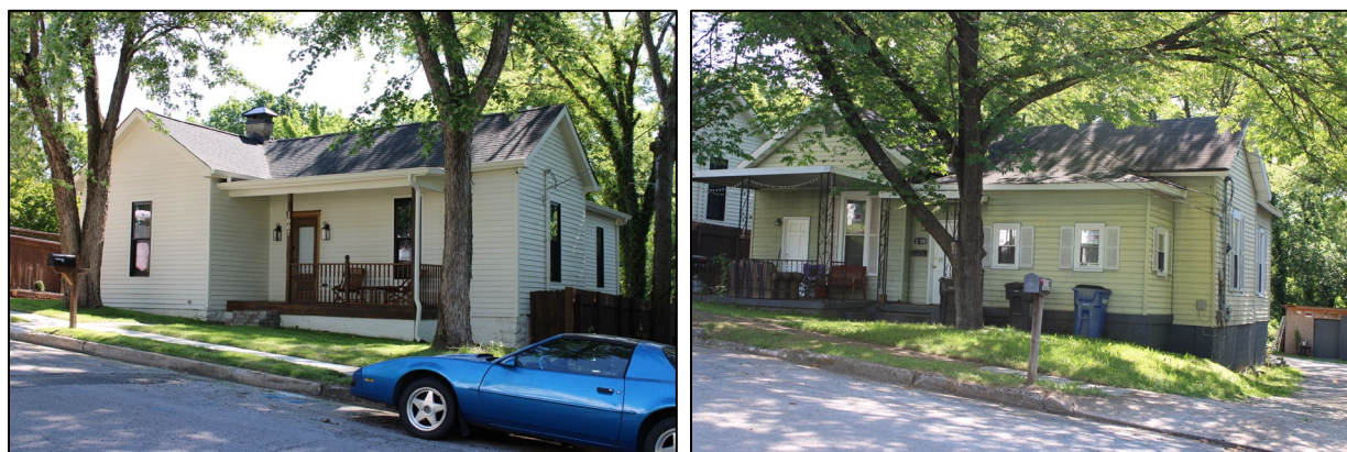
Figure 7-42. Left Photo of Field No. HS-475; view to the northeast. Right Photo of the Field No. HS-477; view to the northeast.
