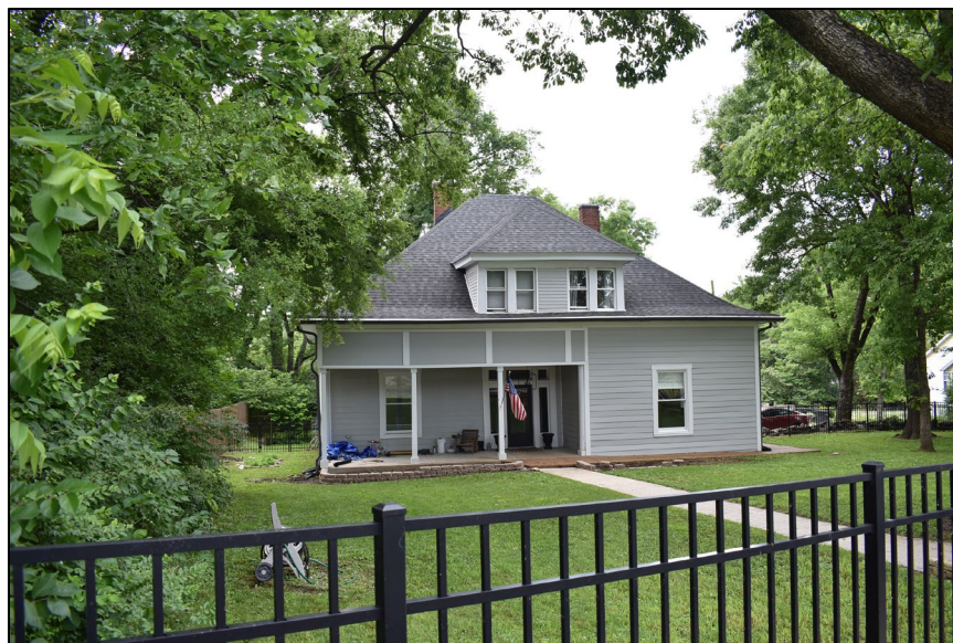
Figure 6-11. Photo of the north elevation of Field No. BC-1 at 713 Trotwood Avenue; view to the south.
