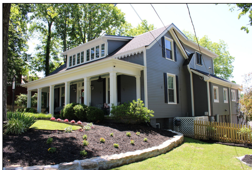
Figure 7-34. Photo of Field No. HS-211; view to the southeast.
