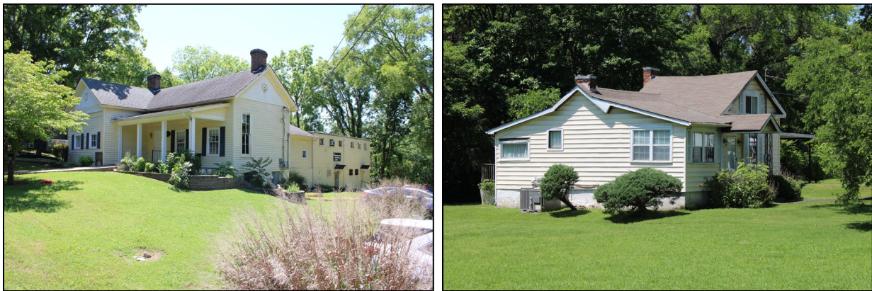
Figure 7-44. Left Photo of Field No. HS-413; view to the southeast. Left Photo of the Field No. HS-513; view to the southwest.
