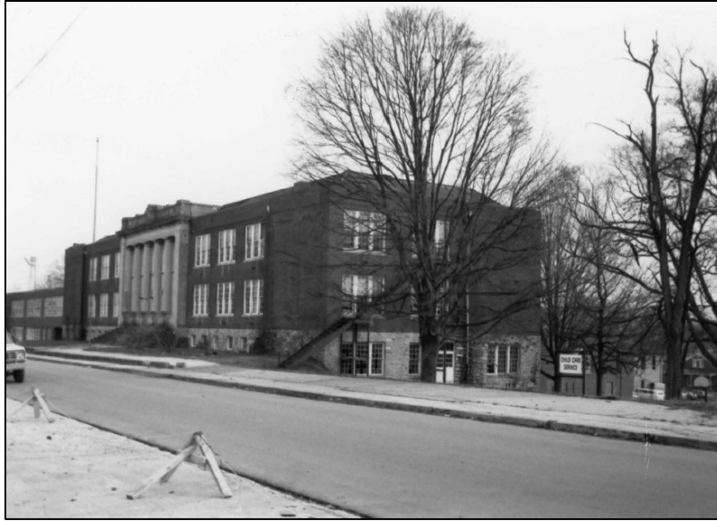
Figure 7-13. D. 1980 photo of d. 1915 Columbia Central High School (Courtesy of NRHP Nomination Form for The Athenaeum [1980] by Rogers and Toplovich).
