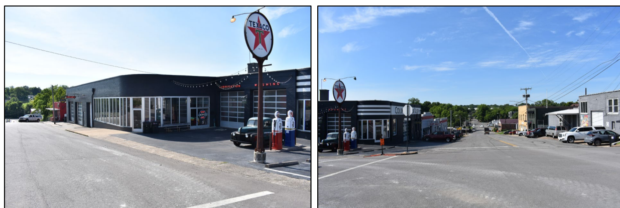
Figure 5-43. Left photo of the Dowling Chevrolet Company Auto Sales & Service Station (Field No. HS-398) and Akin's Market (Field No. HS-224); view to the southeast. Right photo shows Woodland Street between E. 7 th and E. 8 th Streets; view to the south.
