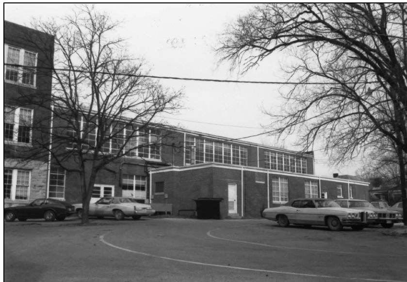
Figure 7-14. D. 1980 photo of d. 1956 Columbia Central High School Cafeteria wing (Courtesy of NRHP Nomination Form for The Athenaeum [1980] by Rogers and Toplovich).
