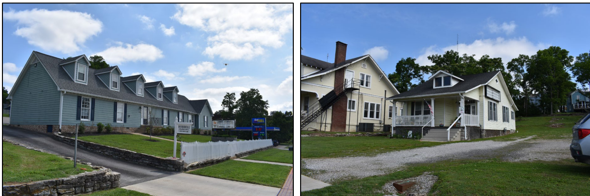
Figure 3-14. Left photo of Redman-David Insurance (Field No. HS-130; left) and Mini Mart (Field No. HS-127; far right); view to the northeast. Right photo of the James Springer House and William Carlton House (Field Nos. HS-130 and HS-133; left to right); view to the northwest.
