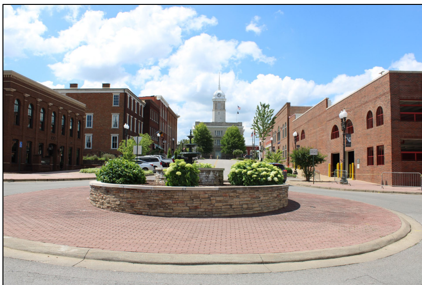
Figure 5-41. Photo of N. Main Street from 6 th Street at the north end of the NRHP boundary for Columbia Commercial Historic District showing Field No. HS-260 (left) and Field Nos. HS-262 and HS-264 (right) outside of the NRHP boundary; view to the south.
