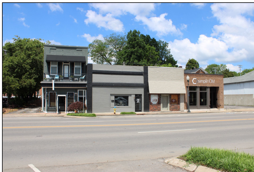
Figure 5-49. Photo of Field Nos. HS-244, HS-247, HS-248, and HS-249 on the west side of N. Garden Street; view west.
