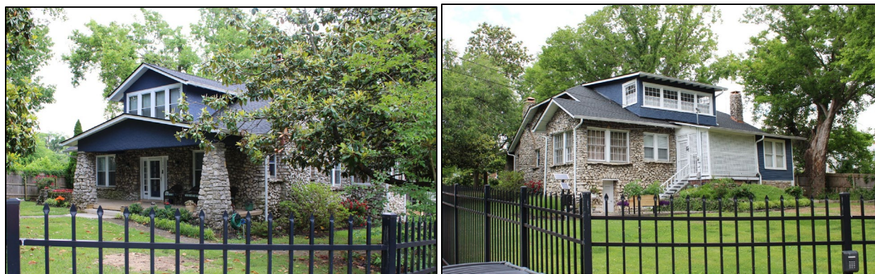
Figure 6-07. Photos of the Mary Harris Barrow House (Field No. BC-2). Left photo shows north and west elevations, and right photo shows west and south elevations.
