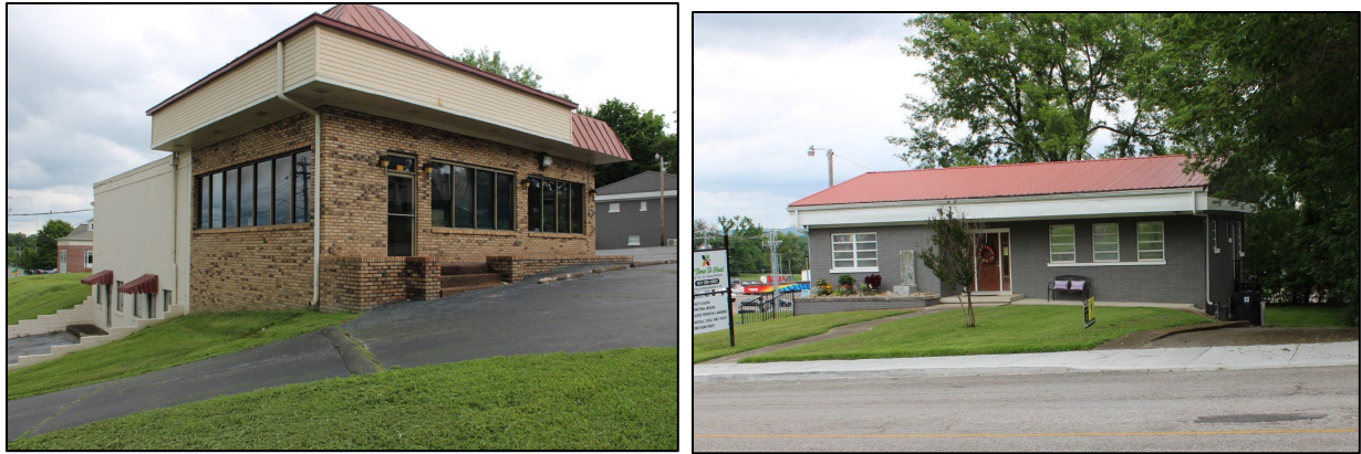
Figure 4-27. Photos showing 600 N. High Street (Field No. HS-80; left) and 604 N. High Street (Field No. HS-82; right).
