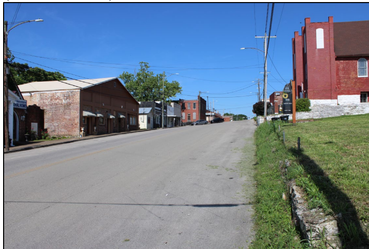
Figure 5-36. Streetscape photo of the southeast side of the NRHP boundary on E. 8 th Street at Woodland Street. This is the historically black commercial area and includes Field Nos. HS-225 to HS-234, and HS-339; view to the west.
