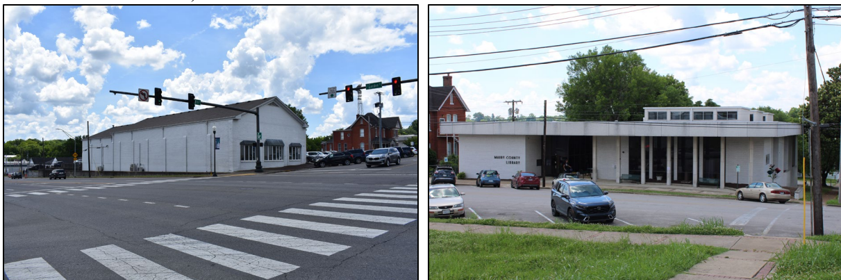
Figure 5-46. Left photo of the south side of W. 8 th Street at S. Garden Street showing Field Nos. HS-386 (left) and HS-387 (far right); view southwest. Right photo on W. 8 th and S. High Streets is showing Field No. HS-389; view to the south.
