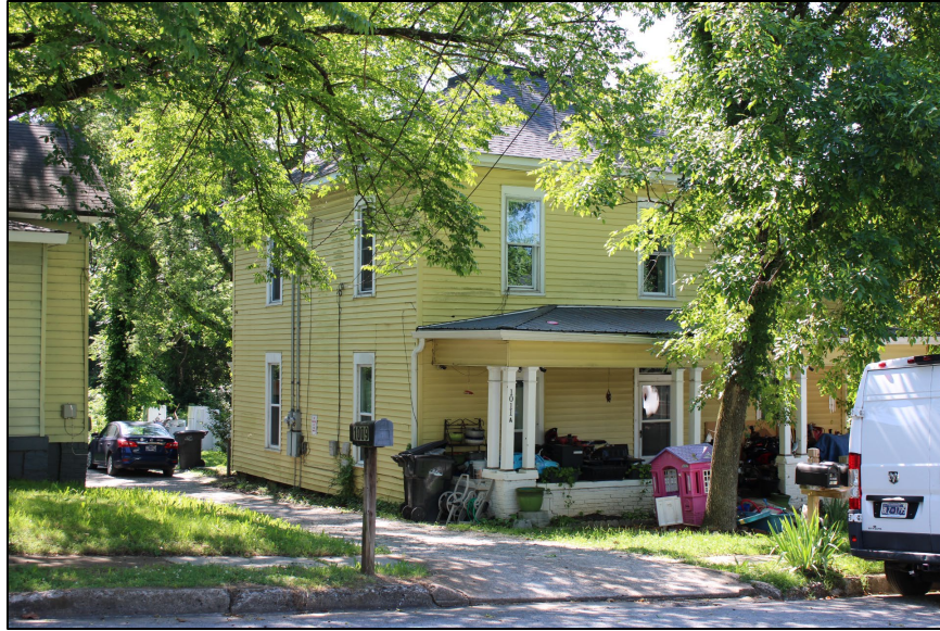
Figure 7-43. Photo of Field No. HS-478; view to the southeast.
