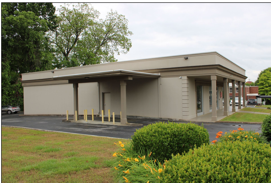
Figure 4-17. Photo of Maury County Federal Savings and Loan Company (Field No. HS-85) at the southeast corner of W. 6 th and N. High Streets; view to the southeast.
