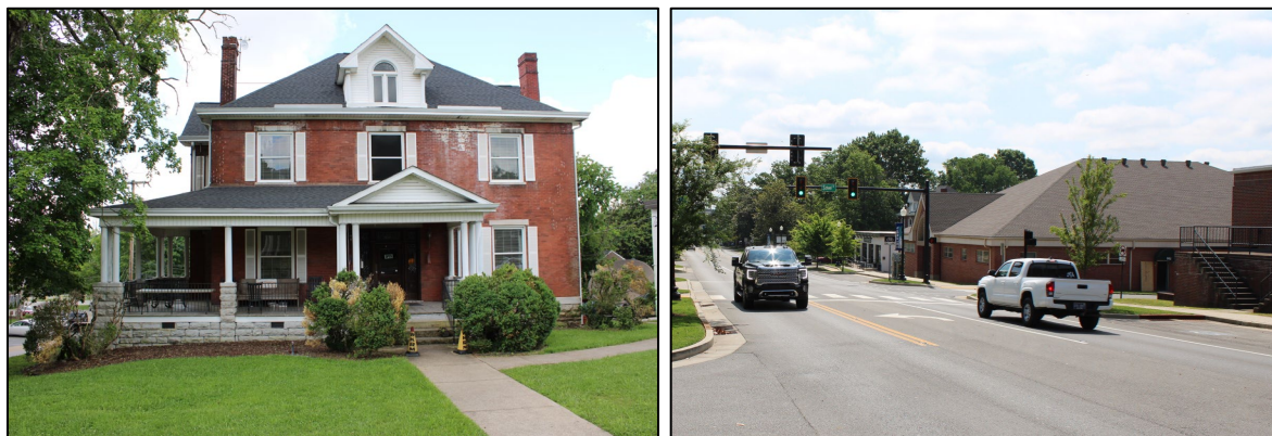
Figure 3-26. Left photo Sparrow House (Field No. HS-120); view south. Right photo on south side of W. 7 th Street between Walker and Athenaeum Streets at Field No. HS-125 and HS-122 (right to left); view to the southeast.
