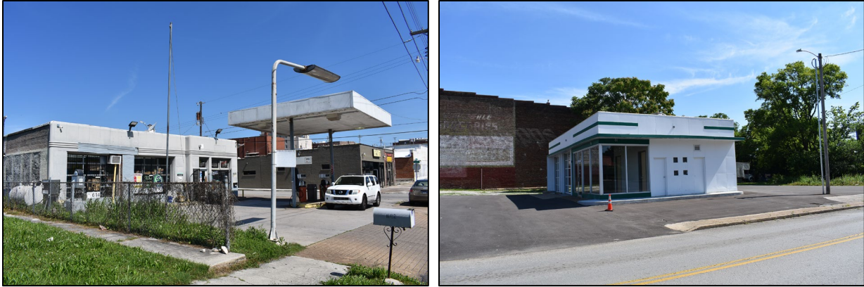
Figure 5-43. Left photo of the c. 1930 Gulf Pride Service Station (Field No. HS-348); view to the northwest. Right photo of the c. 1938 Cathey Tire Company (Field No. HS-347); view to the northeast.
