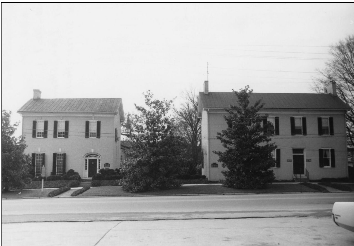
Figure 5-17. 1975 photo of the d. 1816 James K. Polk Home (left) and d. 1818 James Polk's Sister's House (right; courtesy of NRHP Nomination Form for Polk Sister's House [1975] by Cross).
