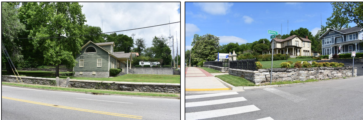
Figure 3-15. Left photo of Gilbert Sister's House (Field No. HS-114); view to the north. Right photo of the Col. Nat. R. Wilkes House and Rev. George Beckett House (Field Nos. HS-141 and HS-140; left to right); view to the northwest.
