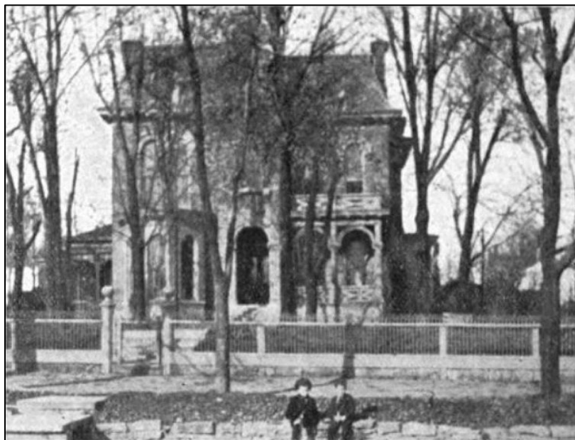
Figure 3-06. C. 1900 Photo of the c. 1873 Church-Barrow House (Field No. HS-119); view to the north (Courtesy of Century Review, 1805-1905, Maury County, Tennessee by David Peter Robbins [1905]).
