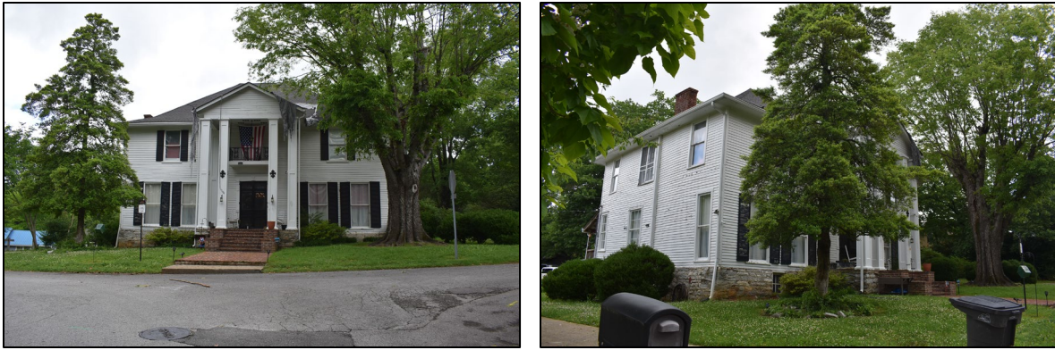
Figure 3-36. Photo of c. 1853 William Wilson House (Field No. HS-96) and c. 1952 Jones House (Field No. HS-95) on Bullock Street; view southwest.
