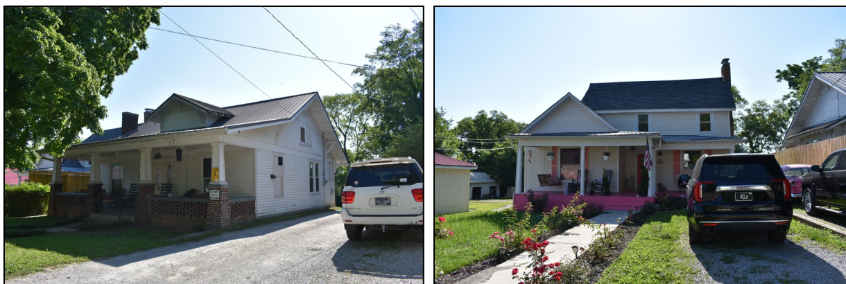
Figure 7-19. Left Photo of the Field Nos. HS-451; view to the northeast. Left Photo Field No. HS-445; view to the southeast.
