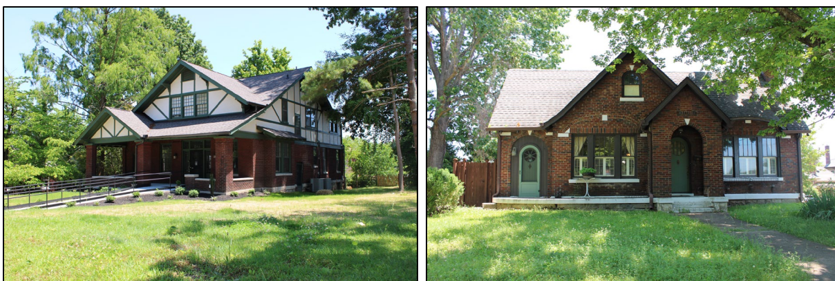
Figure 7-47. Left Photo of Field No. HS-410; view to the southeast. Right Photo of the Field No. HS-412; view to the southwest.
