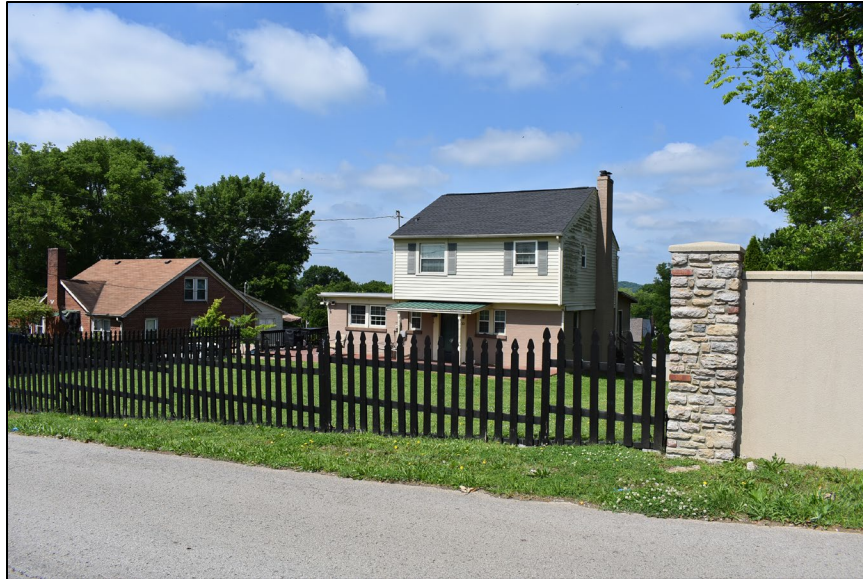
Figure 3-35. Photo of c. 1932 house (Field No. HS-96) and c. 1952 Jones House (Field No. HS-95) on Bullock Street; view southwest.
