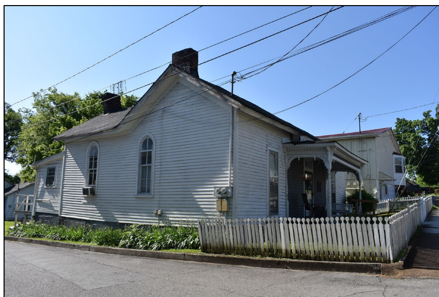
Figure 7-20. Photo of Field No. HS-439 at southeast corner of S. High and W. 10 th Streets with Field No. HS-443 in the right background; view to the southeast.
