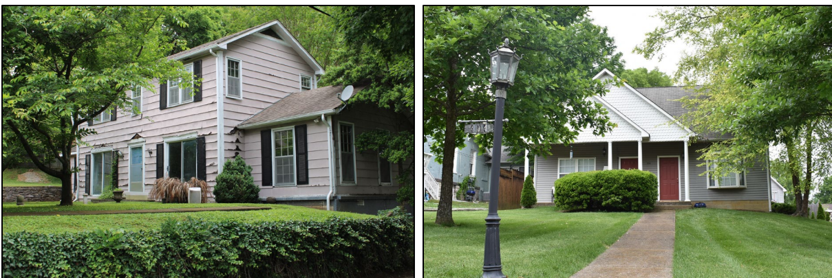
Figure 4-23. Photos showing c. 1979 house at 550 Tulip Drive (Field No. HS-77; left) and c. 1996 duplex at 414 W. 6 th Street (Field No. HS-40; right). Both are infill that do not meet the 50-year criteria and are now considered non-contributing.
