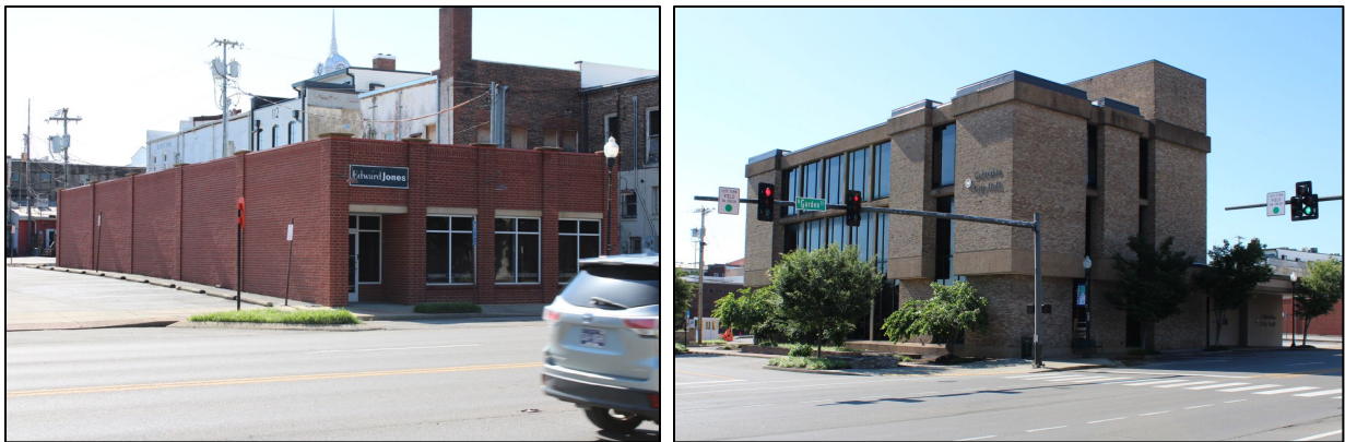
Figure 5-51. Left photo of 710 N. Garden Street (Field No. HS-246); view southeast. Right photo of Middle Tennessee Bank (Field No. HS-241); view to the southeast.
