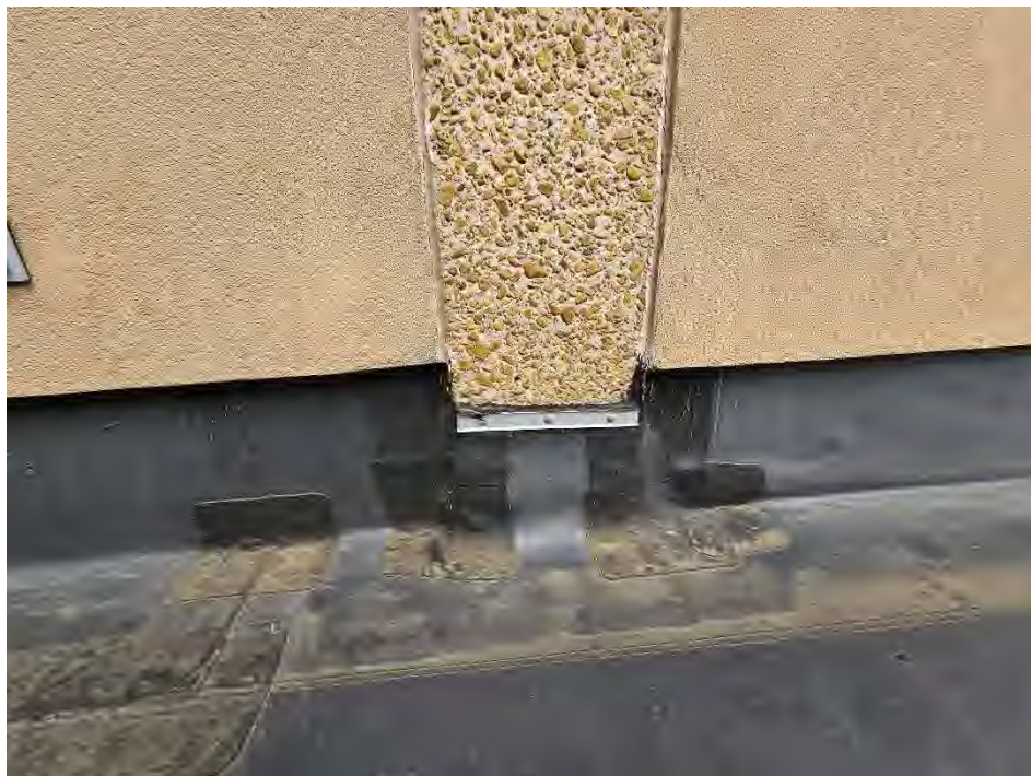
Flashing Detail at the Column
