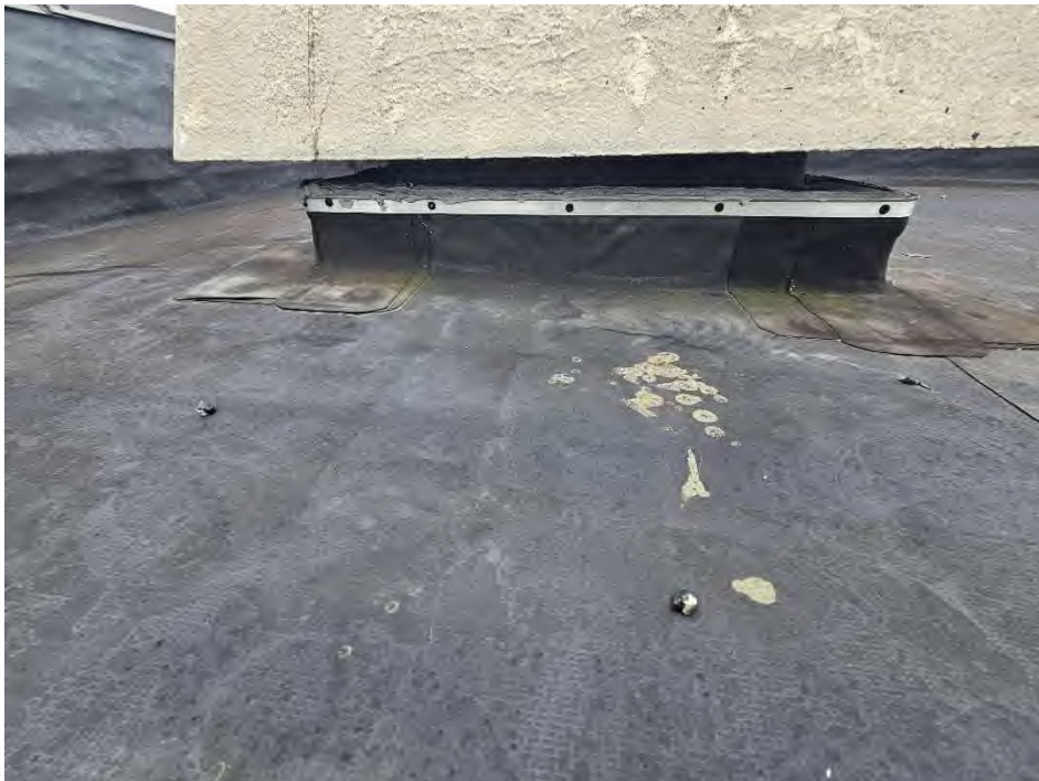
Flashing at Exhaust Fan
