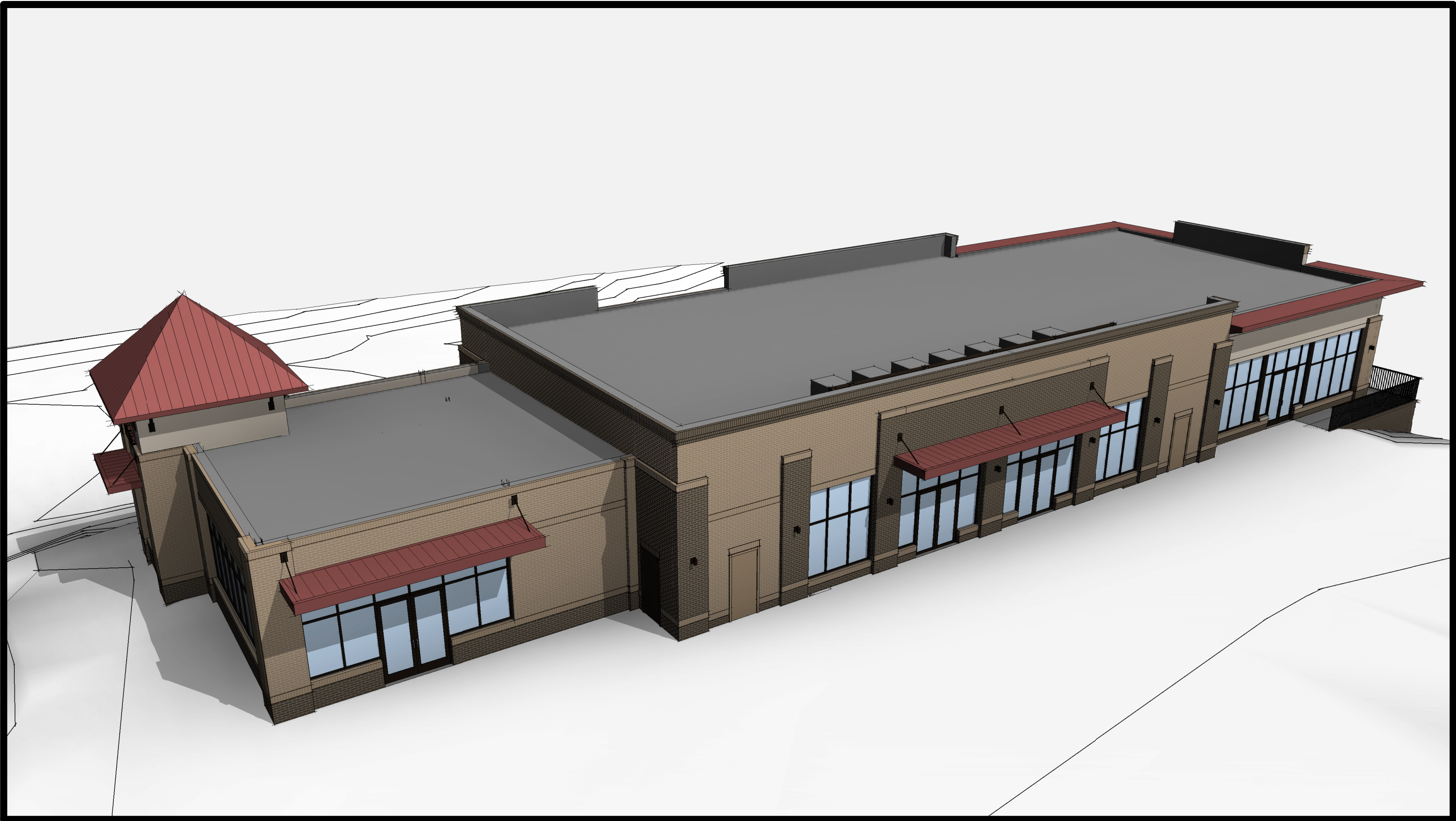
OFFICE + RETAIL - BIRD'S EYE VIEW OF ROOF TOP UNITS BEHIND PARAPET / SCREEN WALL
