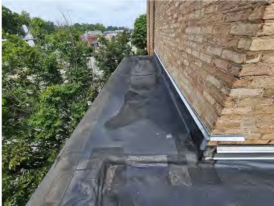
Thru Wall Counterflashing Detail
