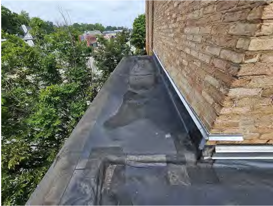
Thru Wall Counterflashing Detail
