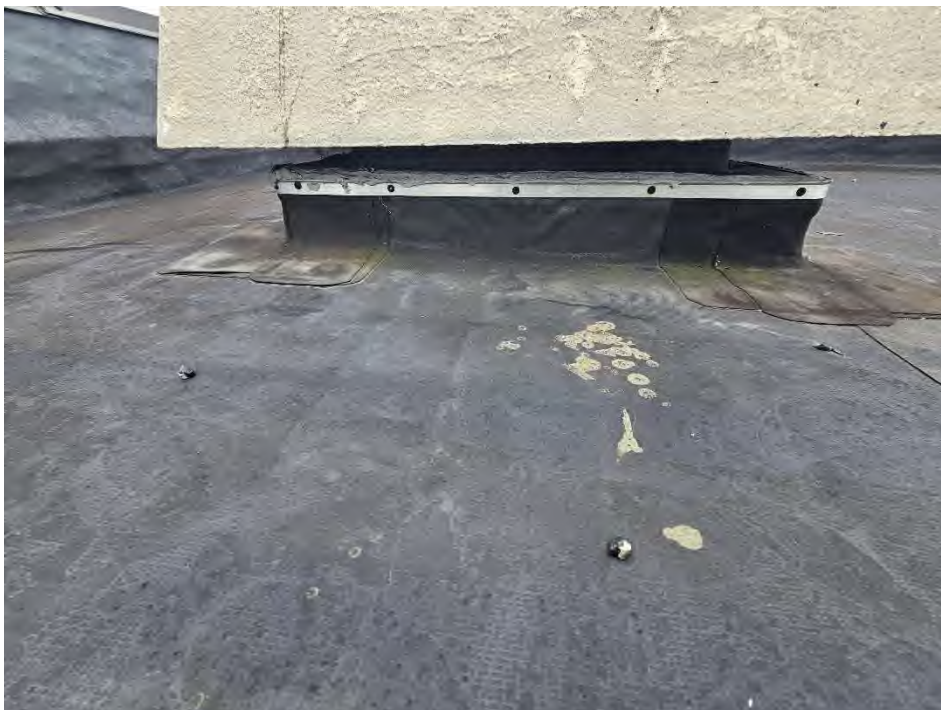
Flashing at Exhaust Fan
