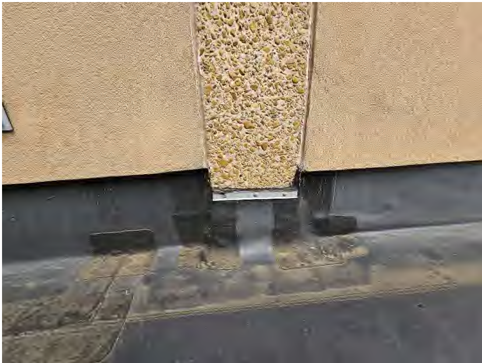
Flashing Detail at the Column
