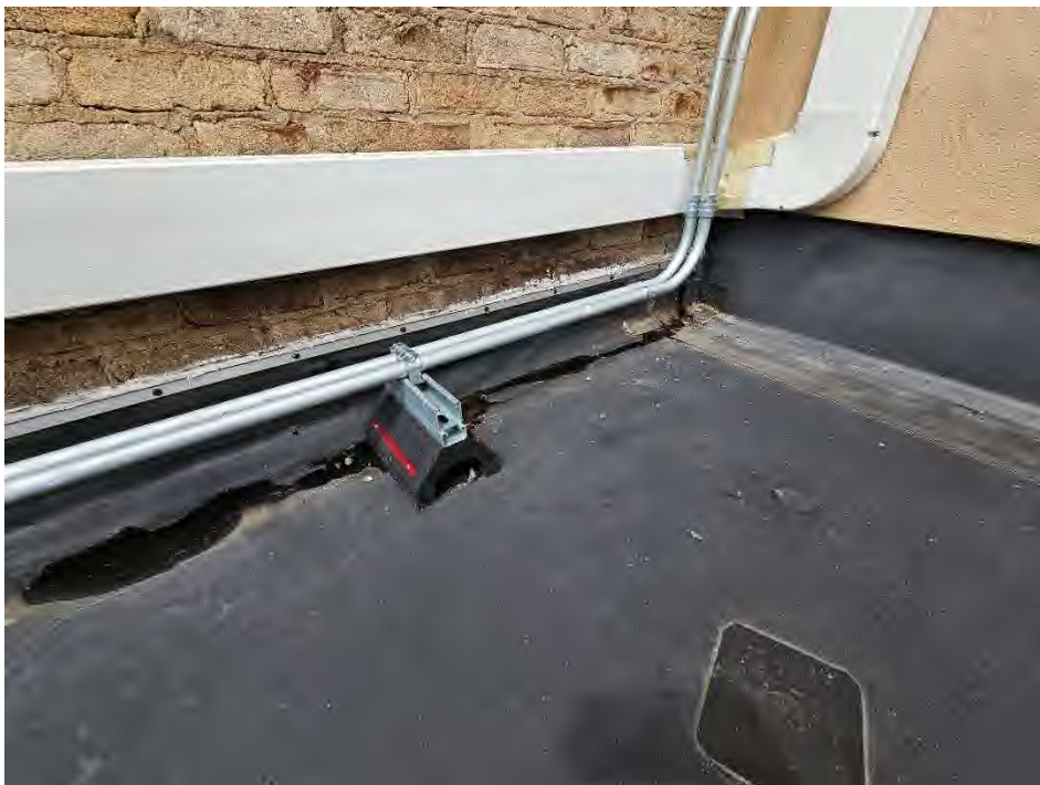
Non-Parapet Wall Detail
