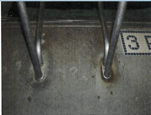
Figure 15 Lap pool ladder grab rails
