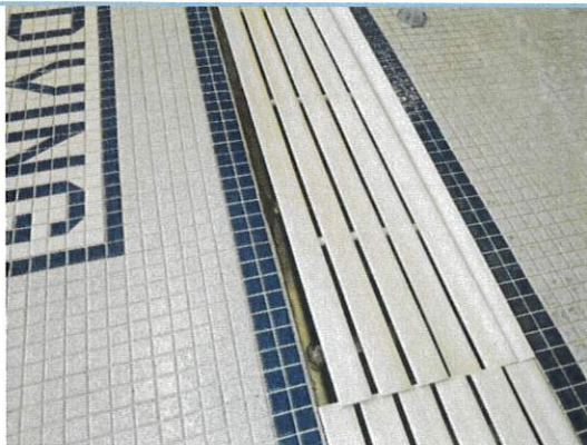
Figure 21 Program pool grating gap
