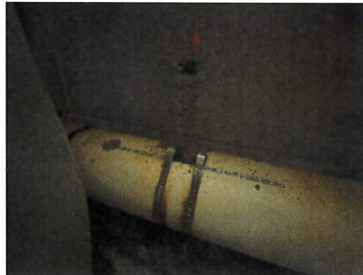
Figure 86 Lap pool flow meter
