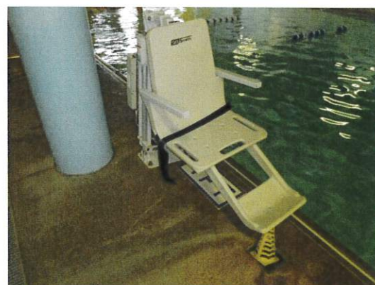
Figure 24 Program pool ADA lift
