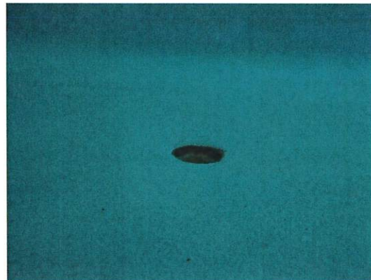
Figure 44 Uncovered pool inlet
