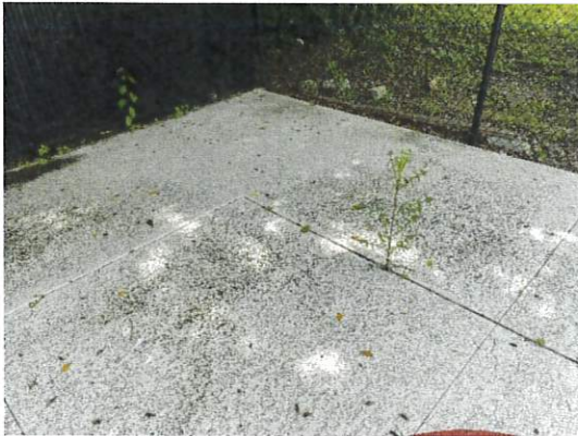
Figure 55 Foliage growing through spraypad deck
