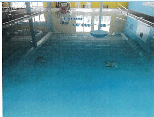
Figure 27 Program pool main drains
