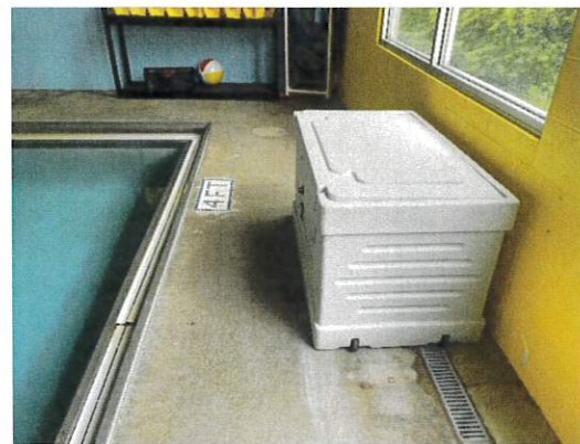
Figure 18 Equipment storage box blocking pool deck circulation
