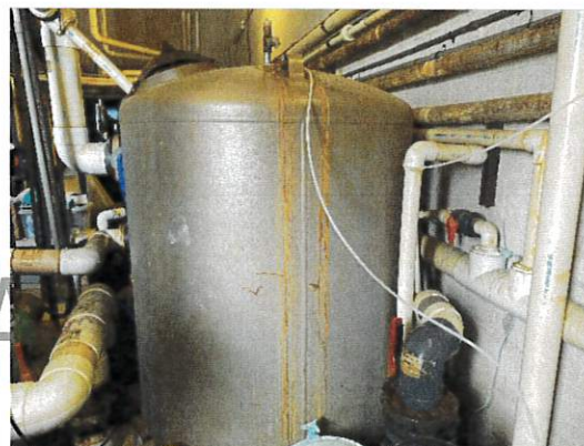
Figure 88 Lap pool chemical feed line
