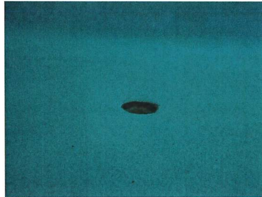
Figure 44 Uncovered pool inlet
