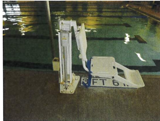
Figure 14 Indoor lap pool ADA lift
