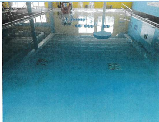
Figure 27 Program pool main drains
