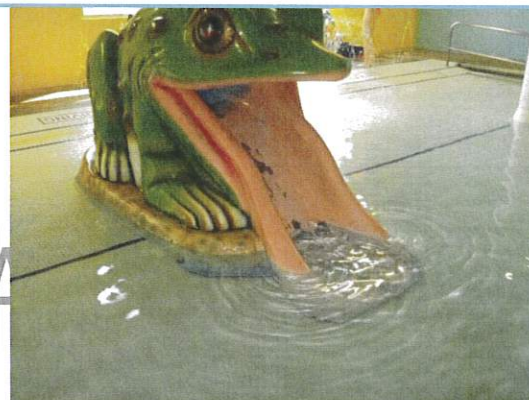
Figure 22 Program pool waterslide (finish coming off)
