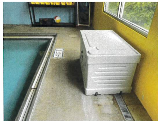
Figure 18 Equipment storage box blocking pool deck circulation
