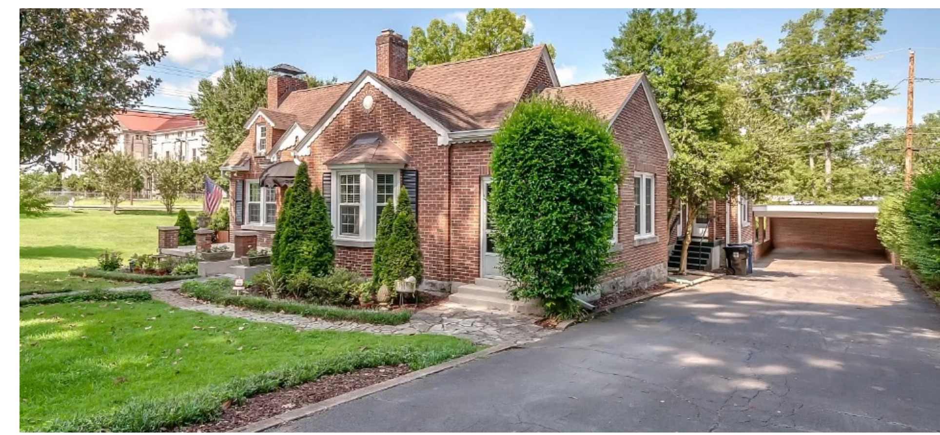
EXISTING HOUSE ON LOT
