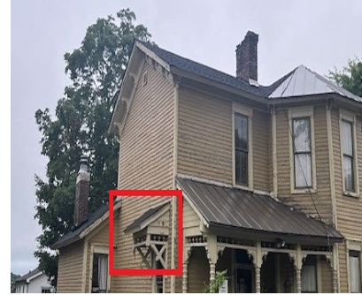
Figure 3 Over stained-glass window east elevation
