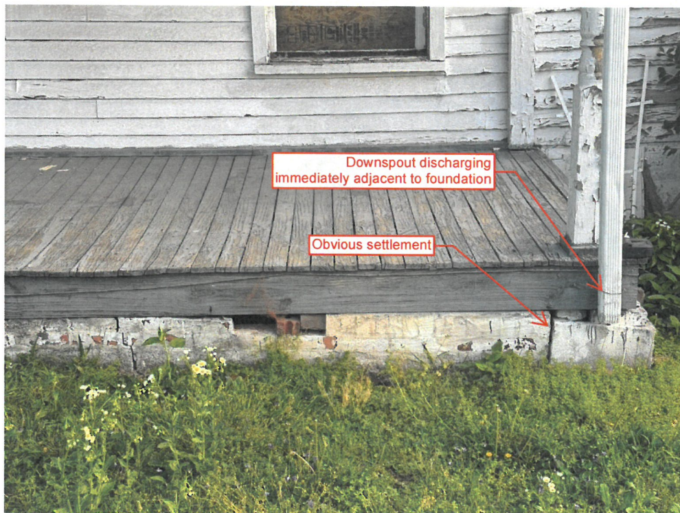
Picture 3: Settlement and Downspout Discharging at Face of Foundation
