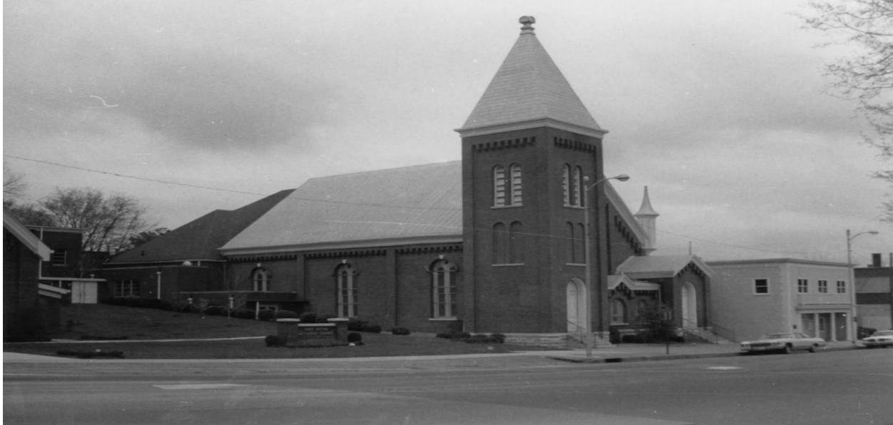
Figure 1 Photo of the First United Methodist Church of Columbia, c. 1984
