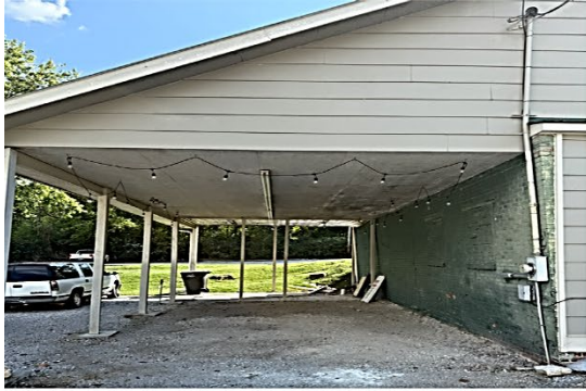
Existing Primary Elevation - Carport Area
