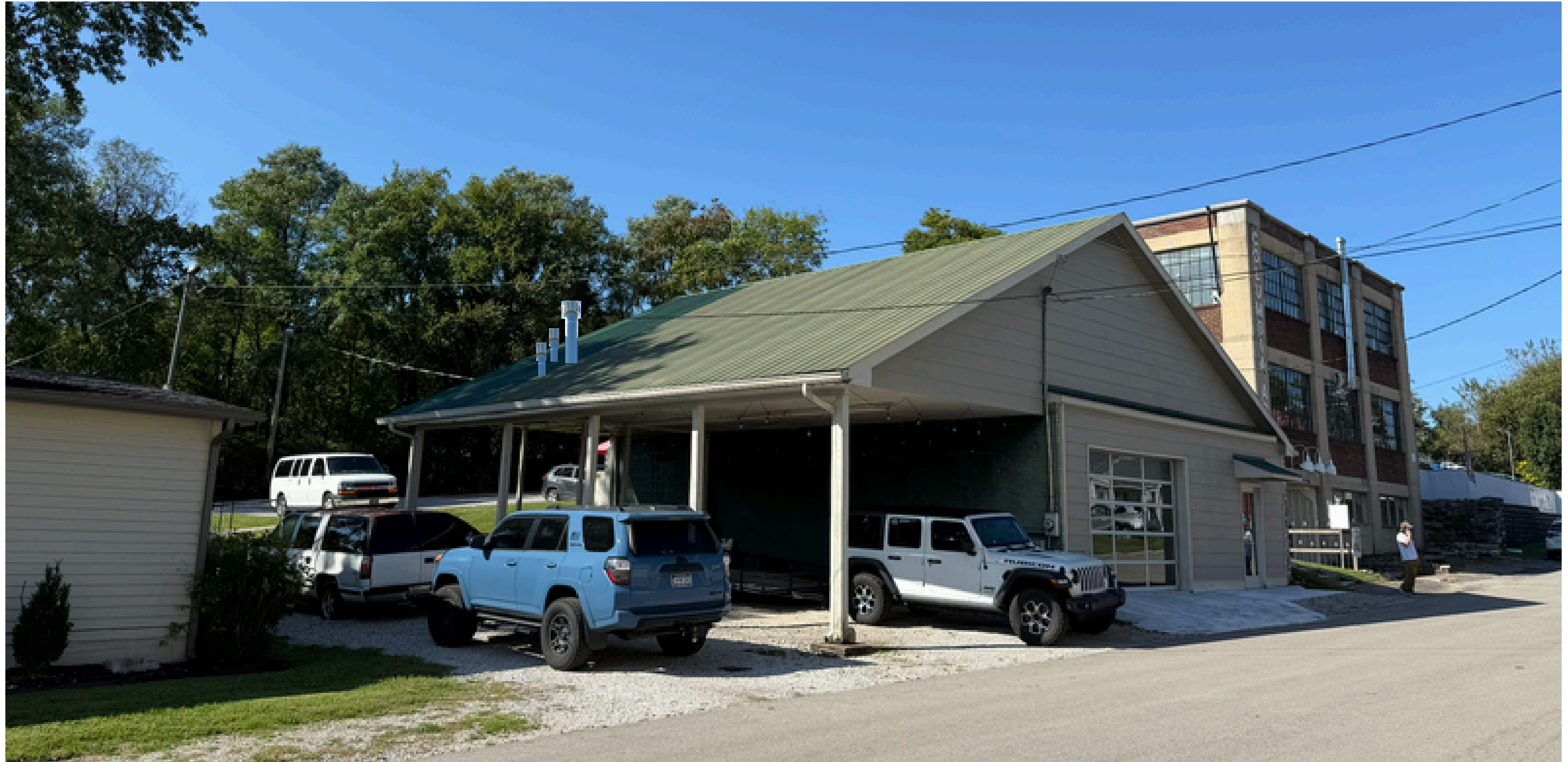
View from S. High Street - shows example of 7' tall 12" boiler vent. Also shows 30" tall 2" return vent, and 30" tall 3" blowdown vent which may not be required depending on final equipment selection.
