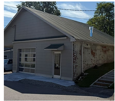
Shown with wall extended to screen boiler equipment in the back of the carport, match existing siding
