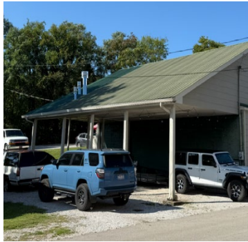
Shown with wall extended to screen boiler equipment in the back of the carport, match existing siding
