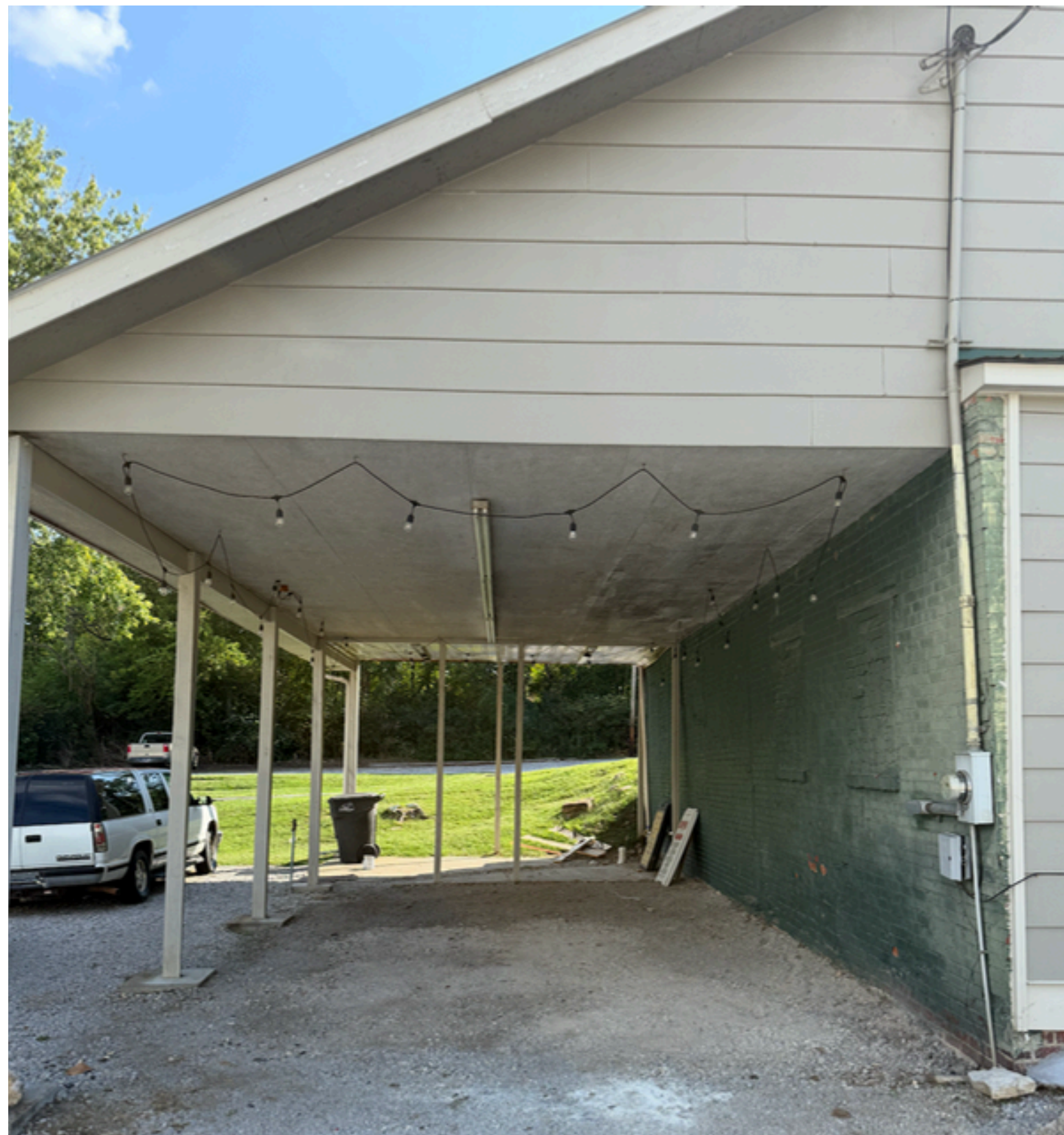
Existing Primary Elevation - Carport Area
