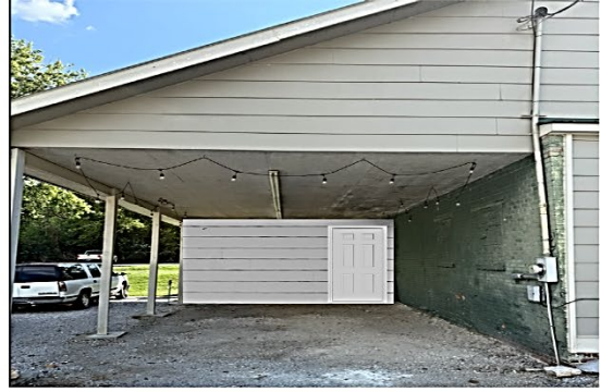
Create walls to match existing siding around the back area. This will shield the new boiler on all 3 exposed sides. There will be 2 fixed louvers on the left wall and a door on the front wall.
