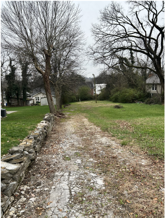
VIEW OF EXITING HISTORIC RETENTION WALL, EXISTING DRIVEWAY, AND BACK OF THE LOT
