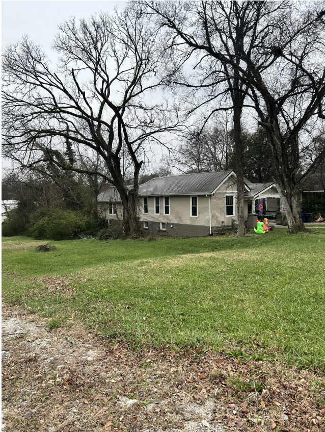
NEIGHBORING HOME TO THE WEST
