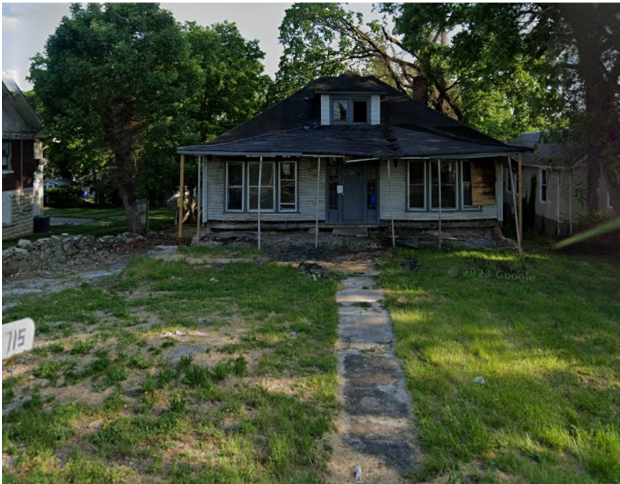
Existing home at 715 W. 7th St, prior to Demolition in 2025
