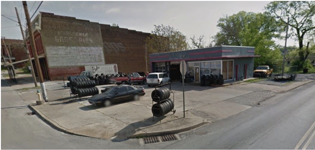
9th & Main, Columbia, TN — prior to renovation
