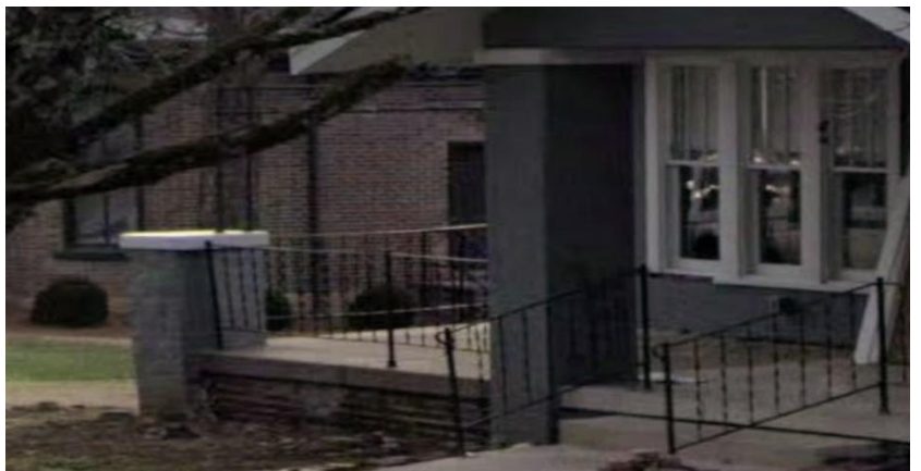
Figure 4 Condition of front porch prior to work
