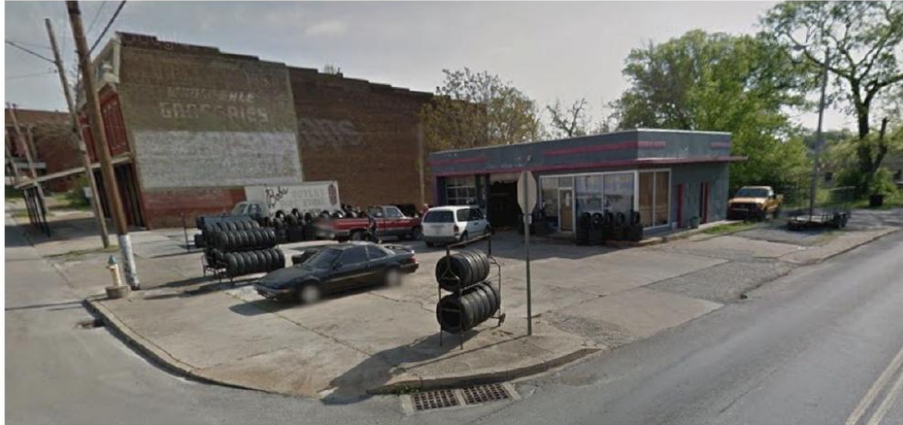
9th & Main, Columbia, TN — prior to renovation
