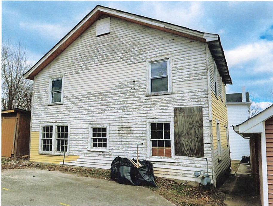
Rear & Side – Southwest Elevation
