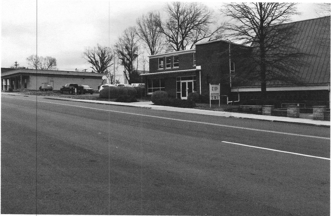
Photo of FUMC Education unit entrance where proposed Canopy would be installed. Photo taken facing North towards the intersection of High street and 6 th St. Building in the background is Multi-Purpose Meeting facility owned by FUMC.
