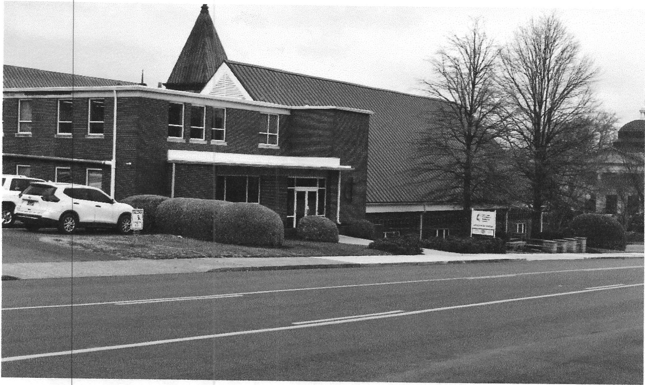
Photo of FUMC Education Unit entrance where proposed canopy is to be installed. This photo taken North of FUMC building facing south towards 7 th street intersection.
