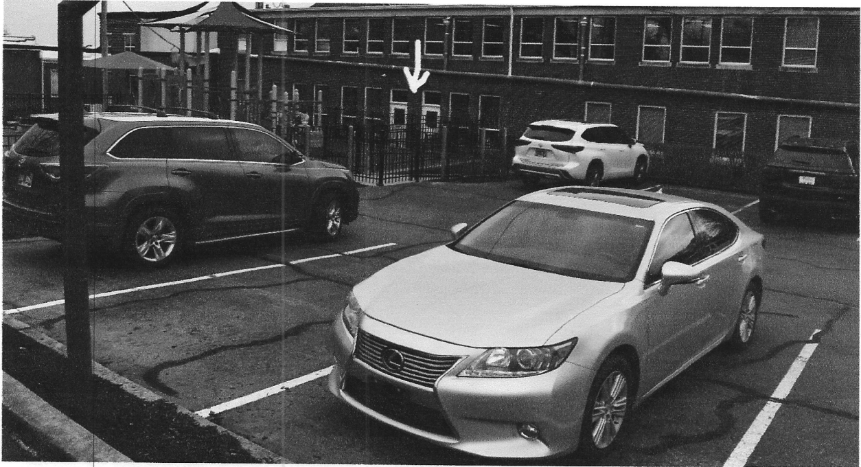
Photo from parking lot of building at 700 North High Street with view of proposed awnings (see arrow) on North wall of FUMC education unit. The building located at 700 North High Street is also owned by FUMC and used as a multi-purpose meeting facility
