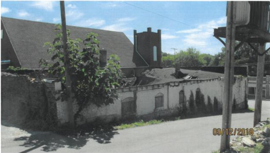
Photo #10: Collapsed roof and damaged walls
