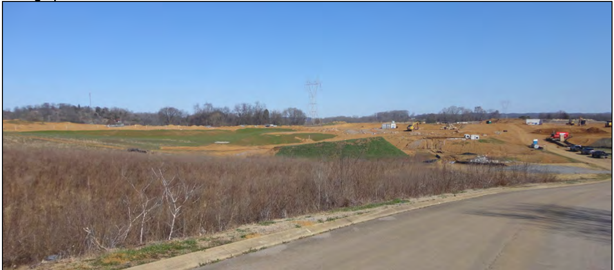
View of tract facing NW from Twin Lakes Drive taken 2/13/2023 by Brandon Malone
