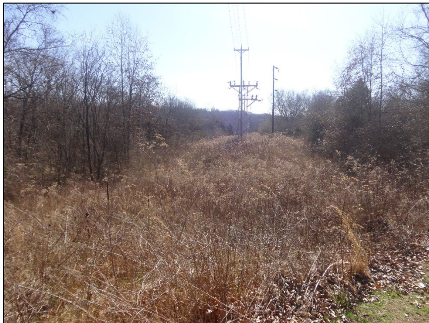
View of electric line easement taken from adjacent tract to the NW facing SE
