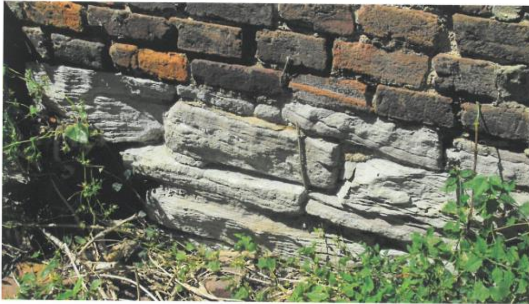
Photo #18: Brick on Stone Foundation
