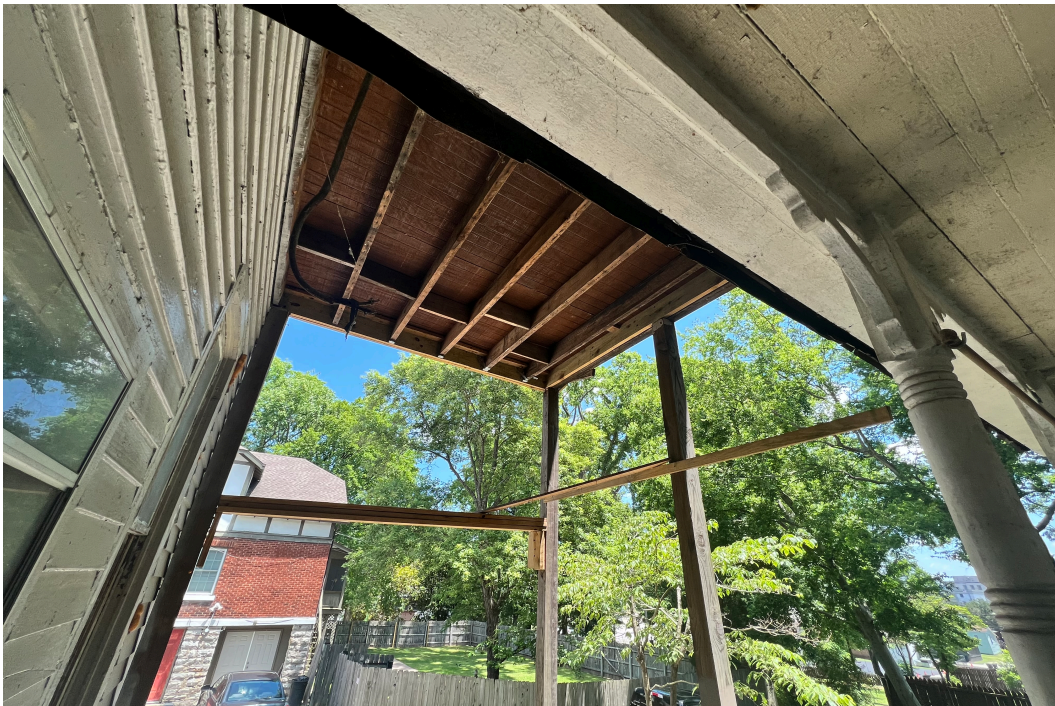
Second story support structure
