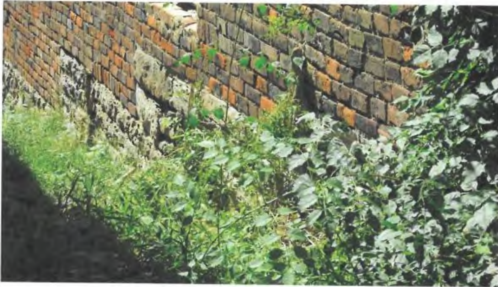
Photo #16: Brick on existing stone foundation on right side
