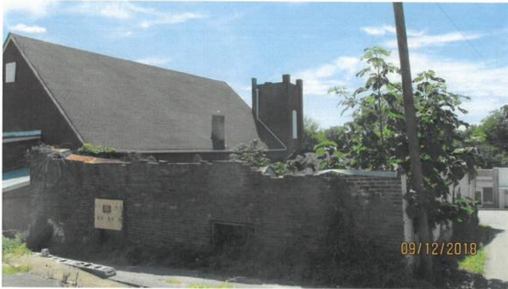
Photo #14: Rear elevation
