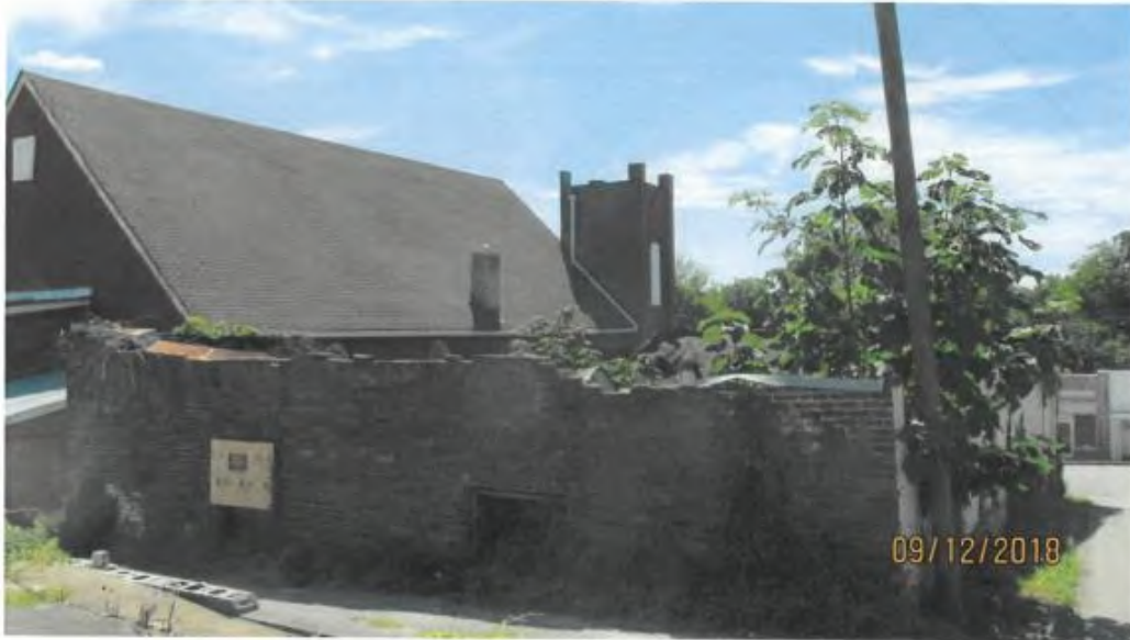
Photo #14: Rear elevation
