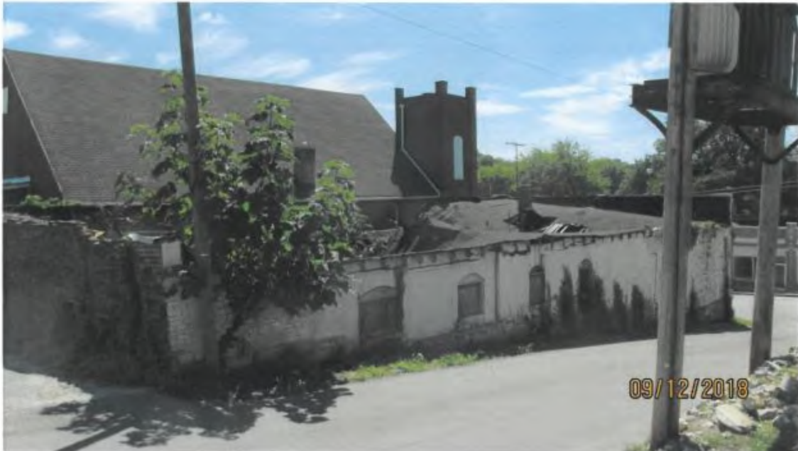
Photo #10: Collapsed roof and damaged walls
