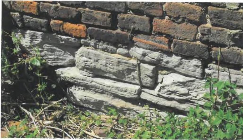
Photo #18: Brick on Stone Foundation
