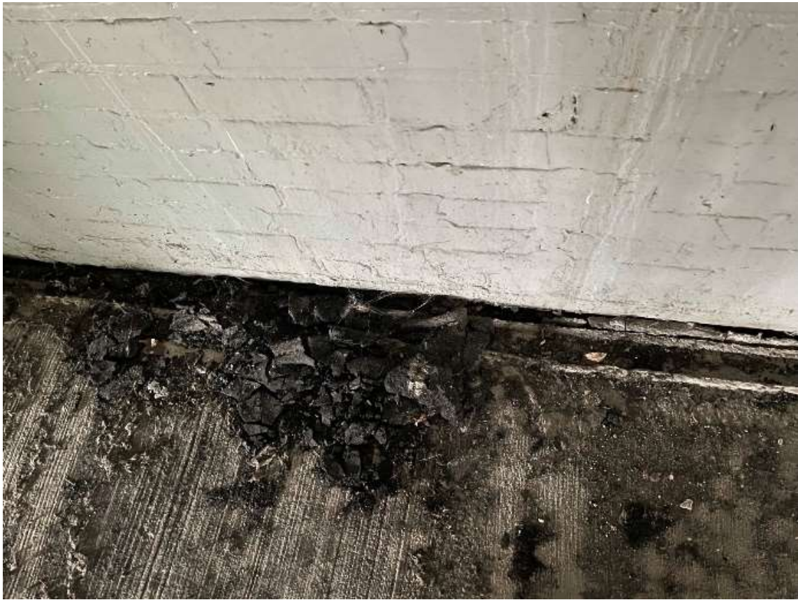
Figure 7 - Expansion joint filler material laying on floor
