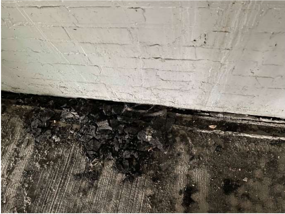
Figure 7 - Expansion joint filler material laying on floor
