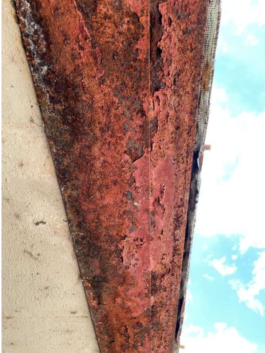
Figure 11 – Corroded lintel
