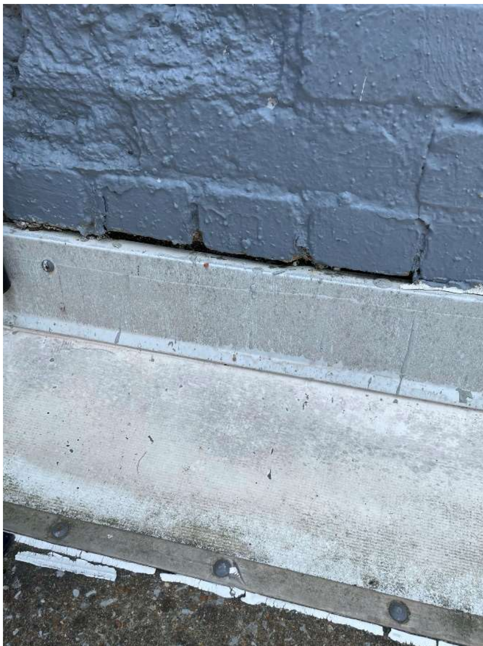
Figure 10 - Brick flashing
