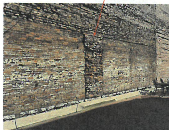
Location where existing infill brick will be removed for new door
