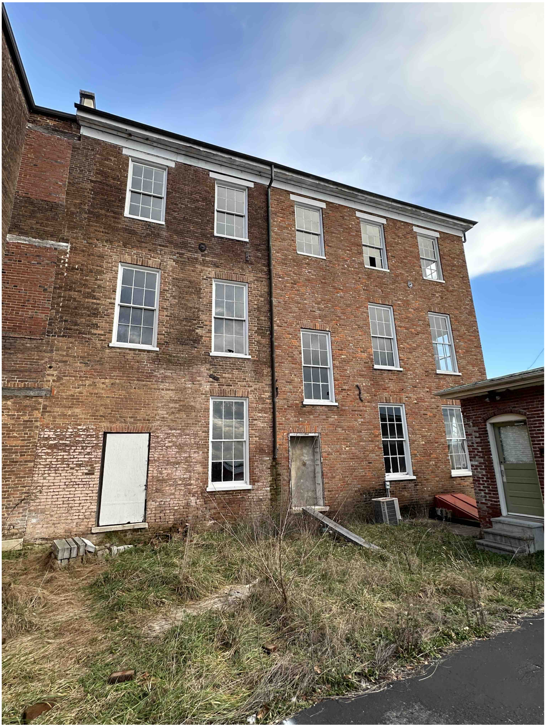
EXISTING CONDITIONS - EAST ELEVATION
