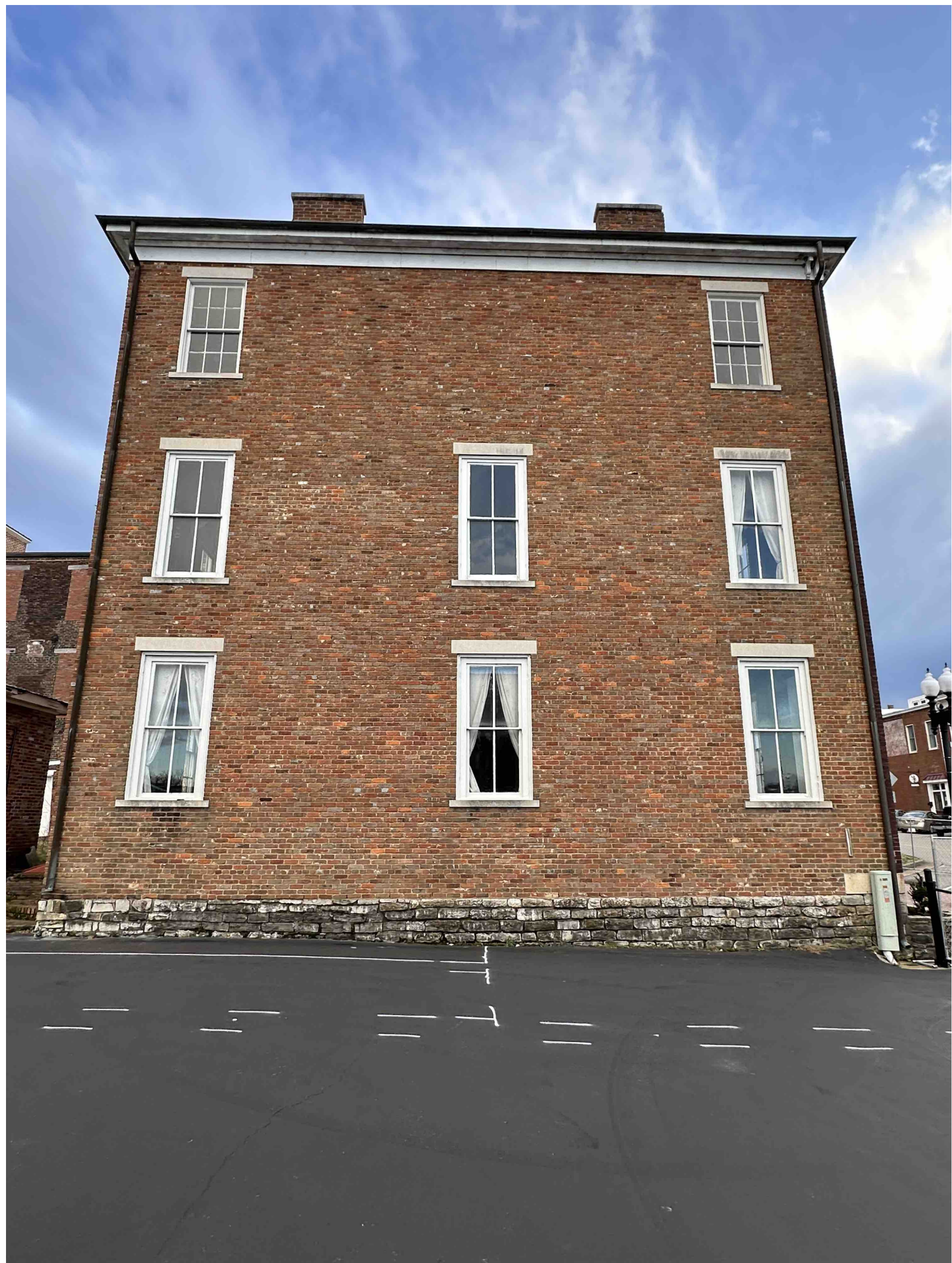
EXISTING CONDITIONS - NORTH ELEVATION
